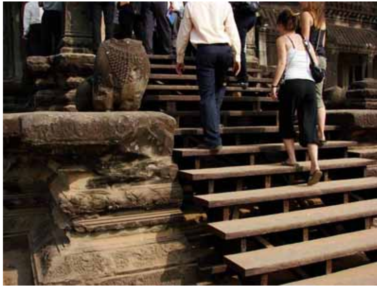
FIGURE 5.5: WOODEN STEPS OVER ORIGINAL STONE STEPS IN ANGKOR WAT, CAMBODIA
